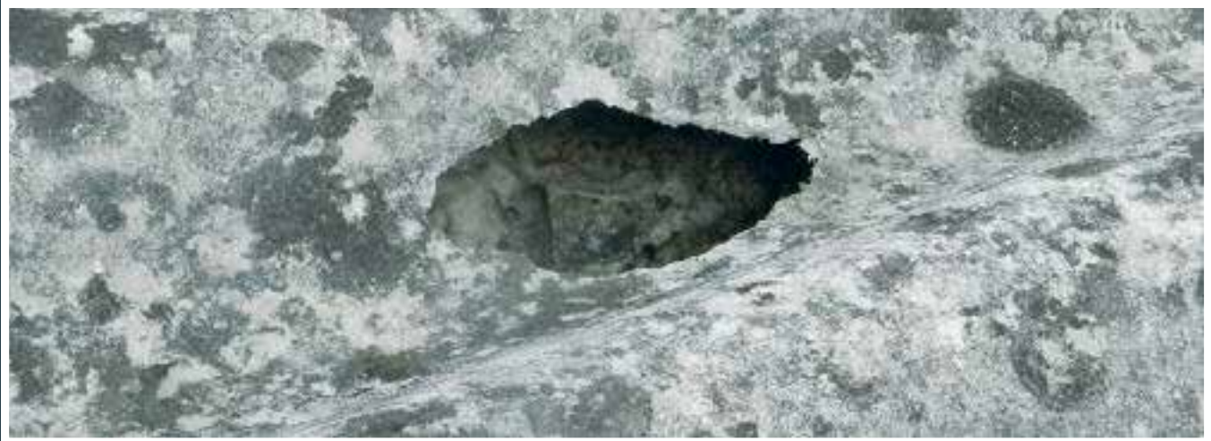
A fibre cement cover clearly broken by hail
