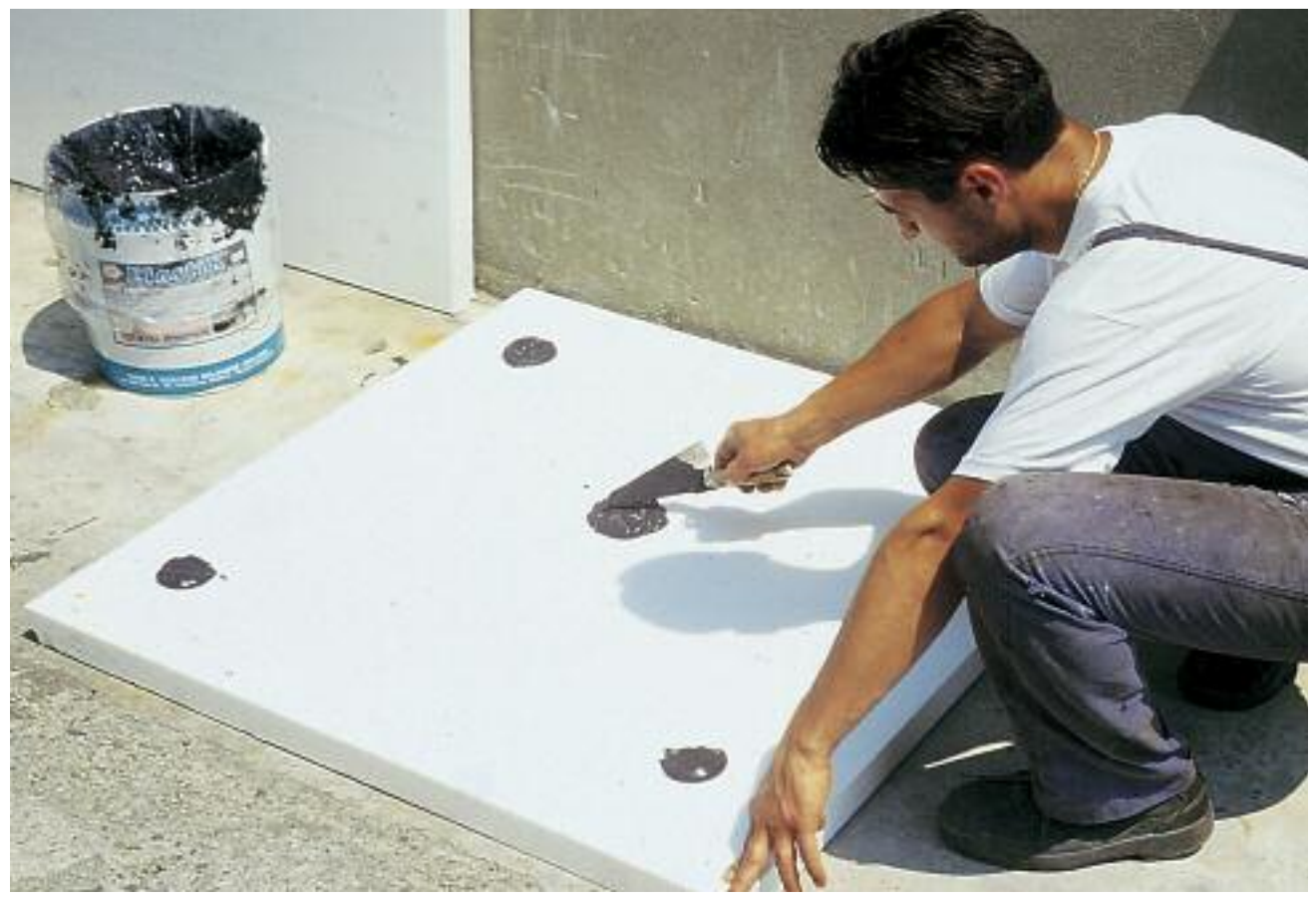
To fix insulated panels to breathable surfaces (ex. concrete, wood)
