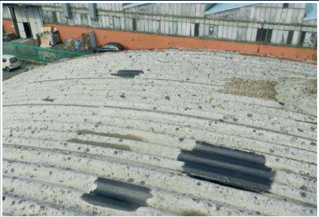
A fibre cement cover clearly broken by hail
