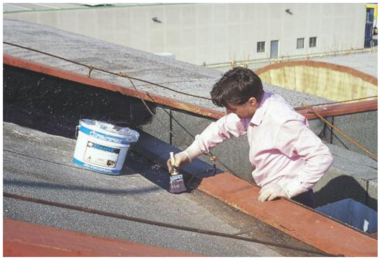
Refurbishments and general maintenance
