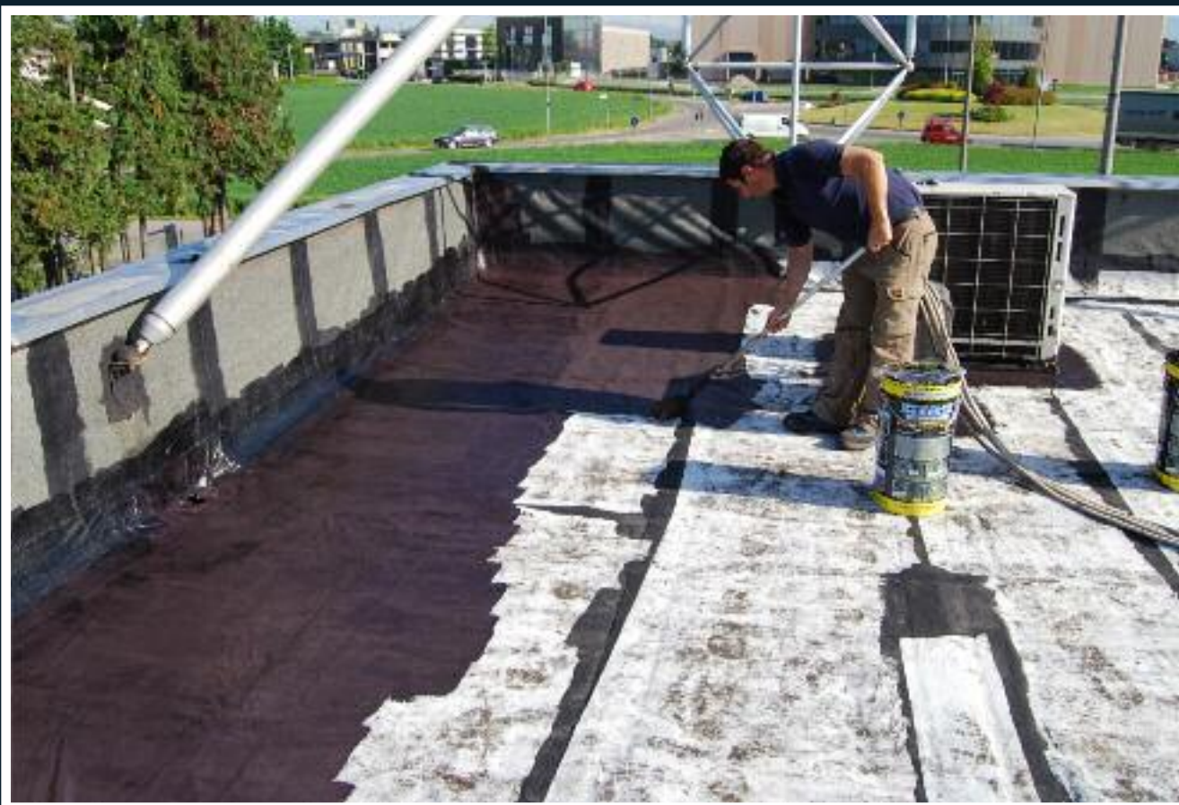
To waterproof the new or repair old bituminous membranes applying ElastiK and Supporto Antifessura (150 g/m 2 polyester non-woven fabric)
